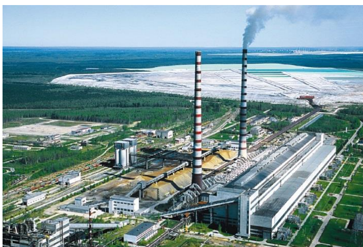
(Photo by Lembit Michelson: Eesti power plant)
