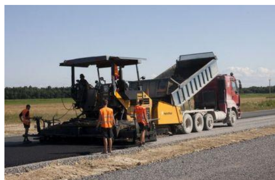
(Photo: Road paving with asphalt; Source: Scanpix)
