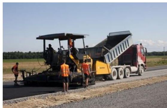
(Photo: Road paving with asphalt; source: Scanpix)
